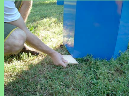
Dealing with uneven ground.
