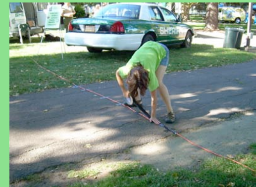
Taping electrical cords.
